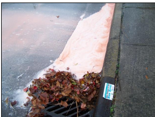
Suspicious color flowing into a storm drain is a good example of illicit discharge coming from some location nearby.
