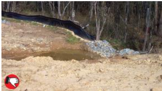
Example of poor trap installation. Overflow notch is too deep and surrounding area needs seed and mulch to prevent erosion.
