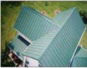
Roofing, Patios, Sidewalks
